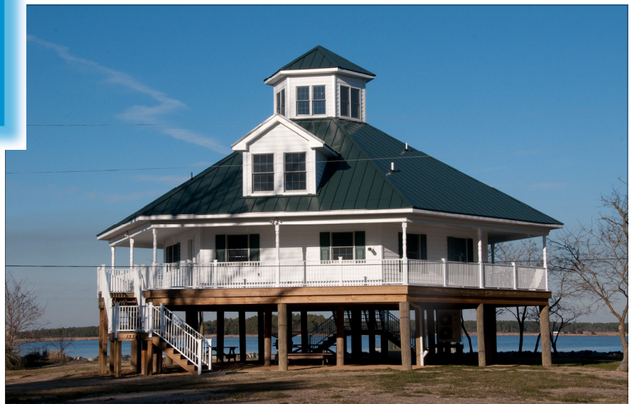
Daikin's flexible heating and air conditioning system gave the architect the freedom to design this amazing replica of the original Hooper Strait Lighthouse.
